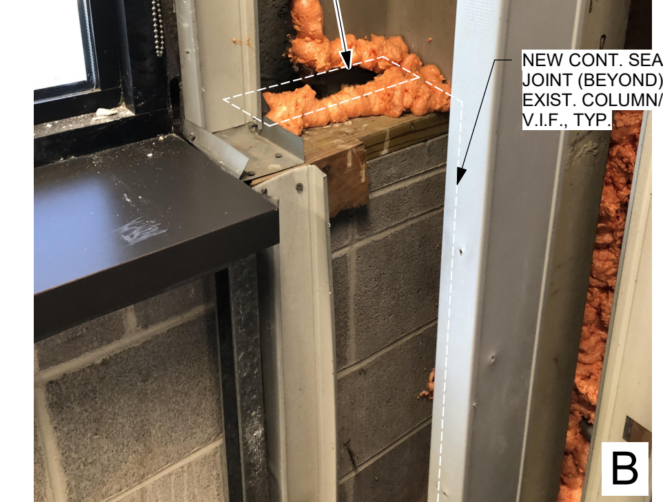
COLUMN/ WALL EXISTING CONDITIONS
